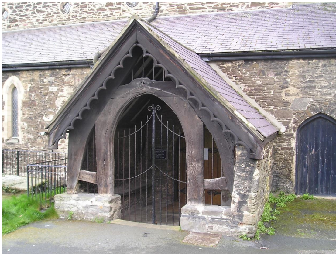
Conwy church porch, Wales.
