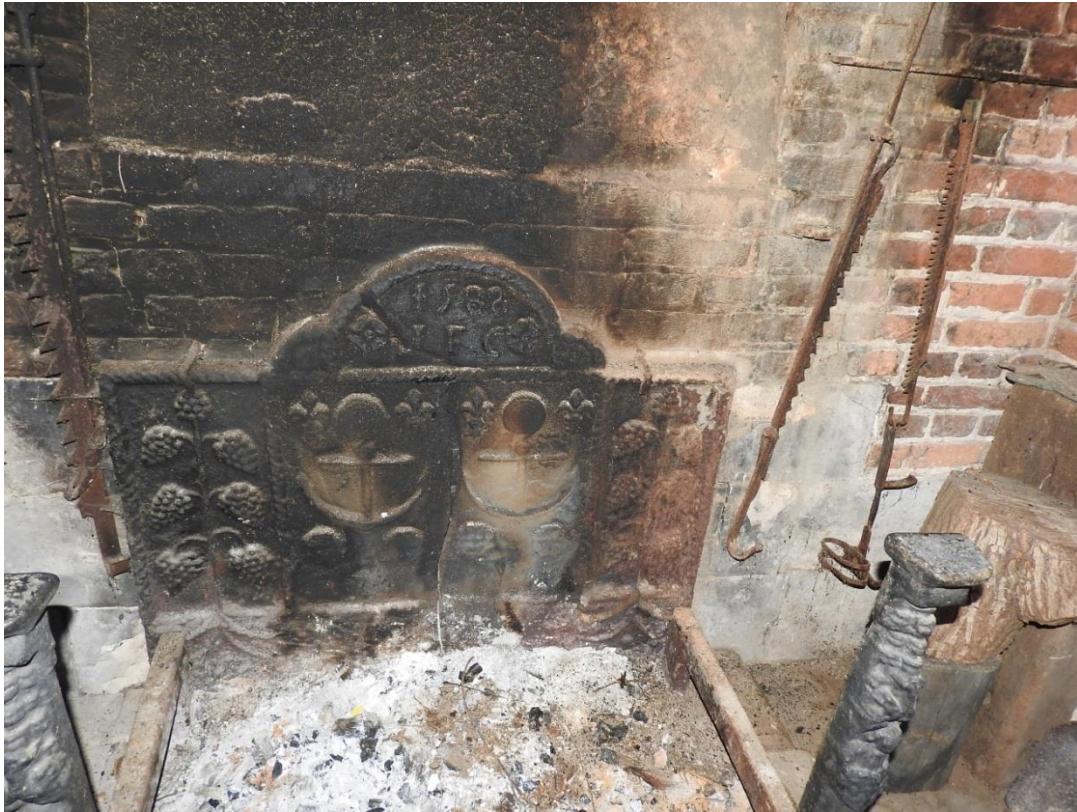
Armada fireback from Nutfield with single side panels, two panels each side were used if a very wide fireback were needed.
