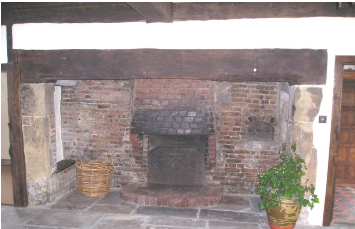
A simple fireback from Godstone with straight lines created from rope twisted around a rod flanked by rose and shield impressions
