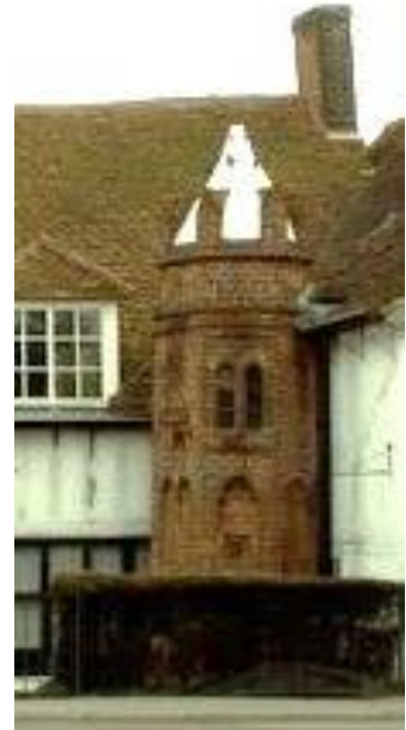
Detail of stair turret
