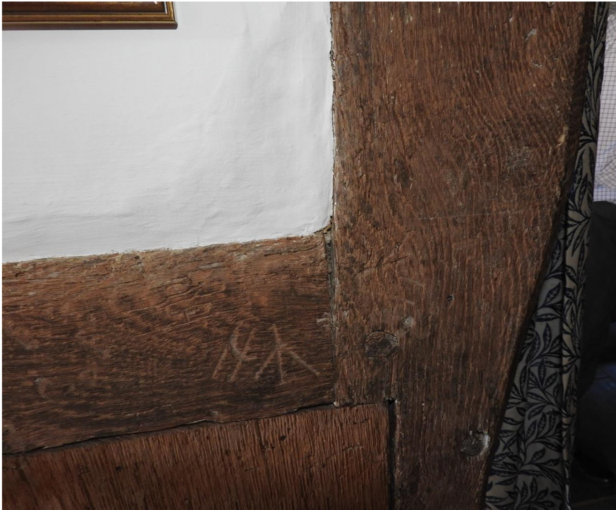
Carpenter's assembly number III with both crow's foot and crescent tags in Nutfield.
