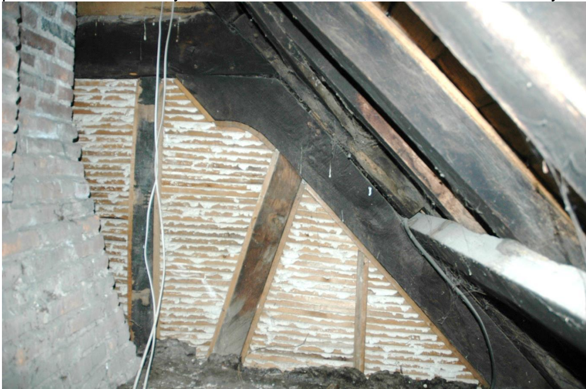
North side of frame C, showing the clasped lower purlin
