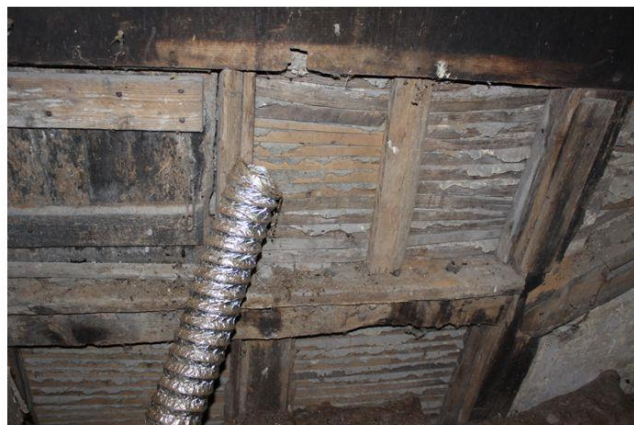
Top. Frame A from south Below. Detail around 'vent'
