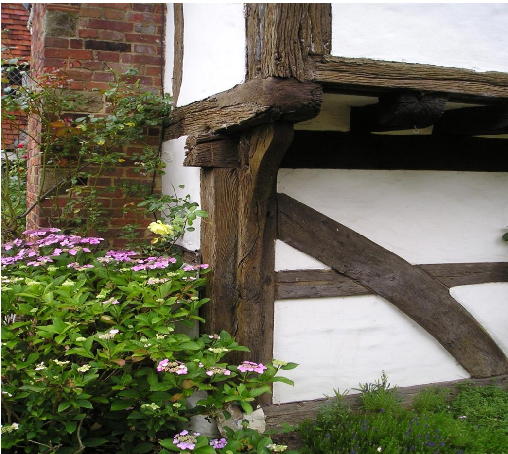
Cogmans, Burstow (1476). Jetty plate bridled to first floor post.
